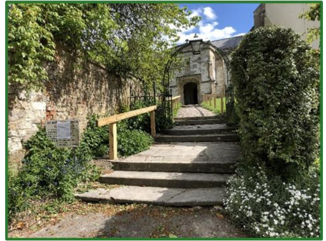
New handrails at St Mary's Ashbury
